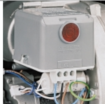
Control box fitted with an ignition transformer
